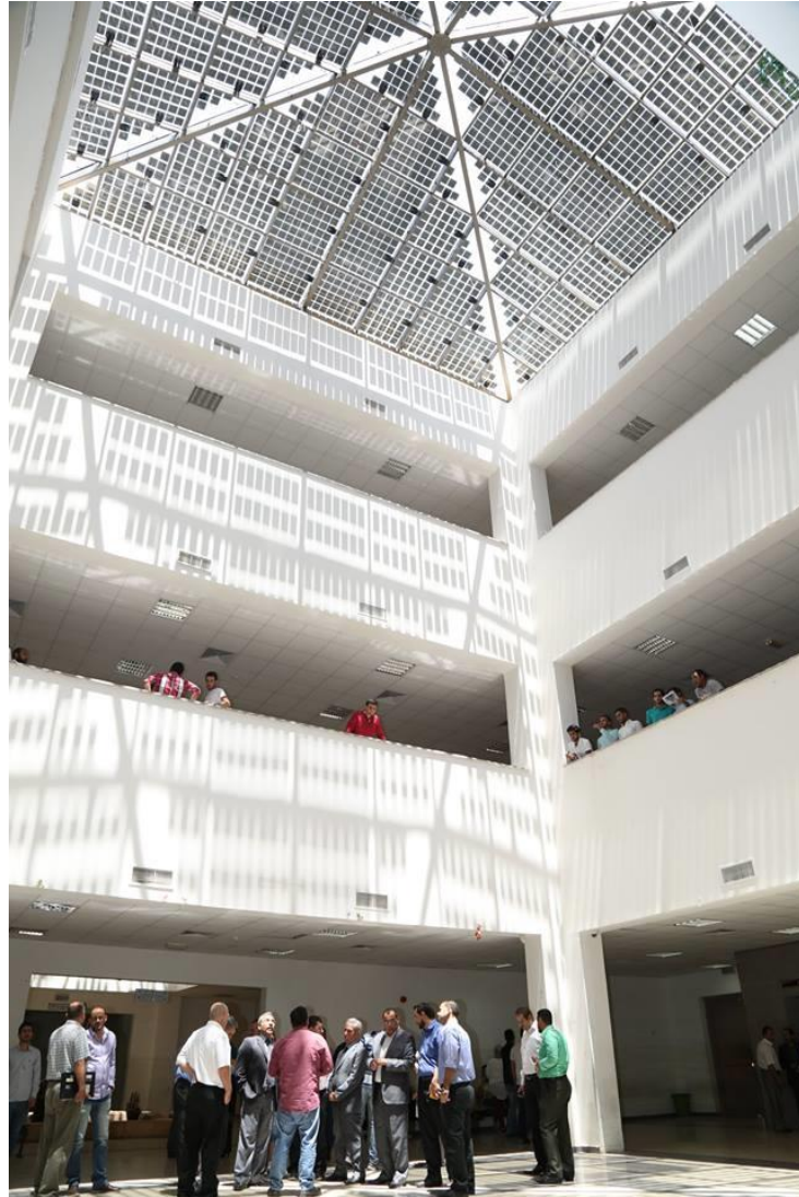
Figure 10 Solar BIPV installed in Aqaba branch.
